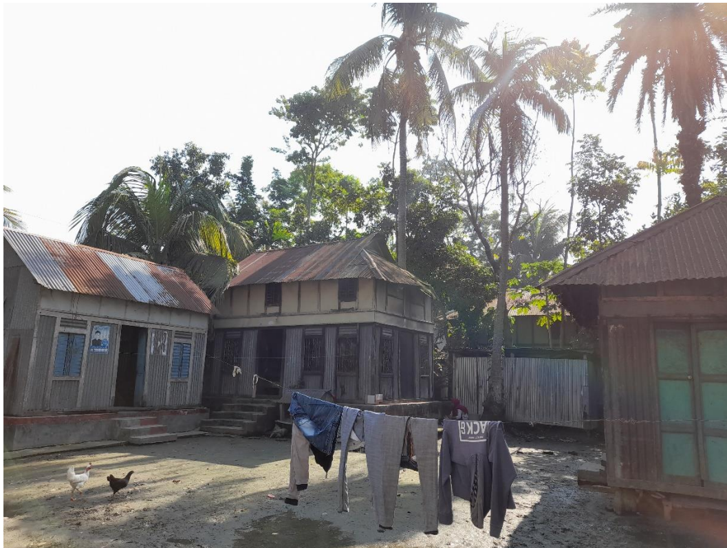
Fig 5.7: Semi-pucca settlements of Mandra (Source: Field Survey 2021)
